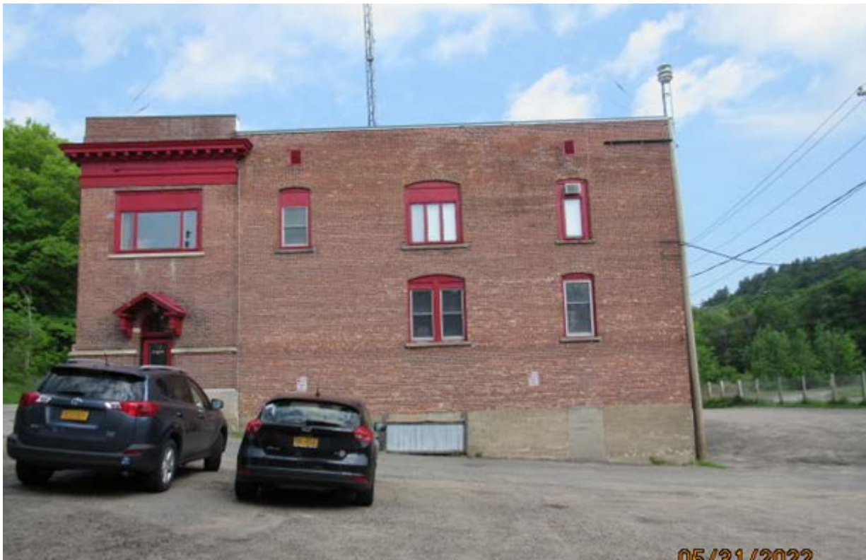
Figure 8: SLVFD side view
