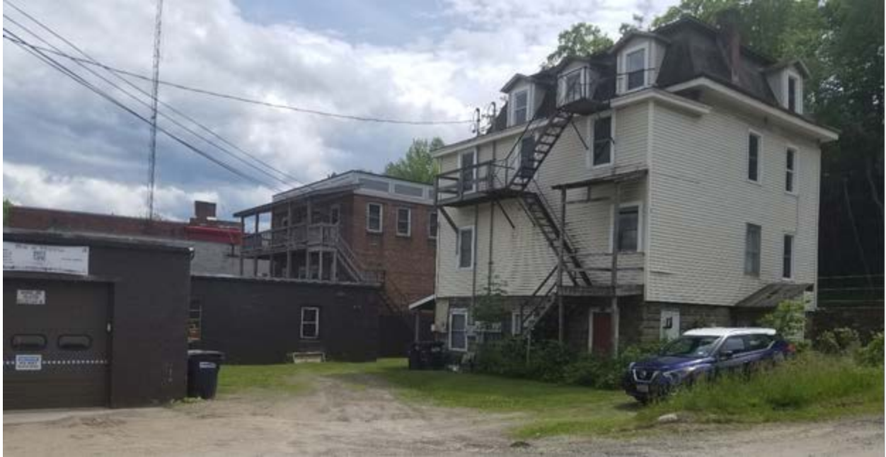
Figure 22: Structure being considered for acquisition by SLVRS
