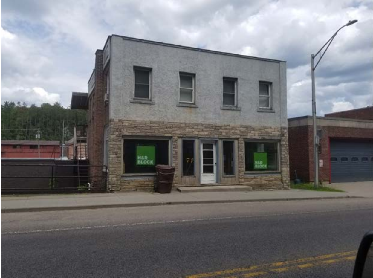
Figure 11: SLVRS front view (sleeping quarters on second floor)
